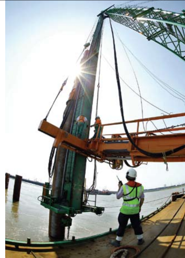
Pile driver working on sea defences
