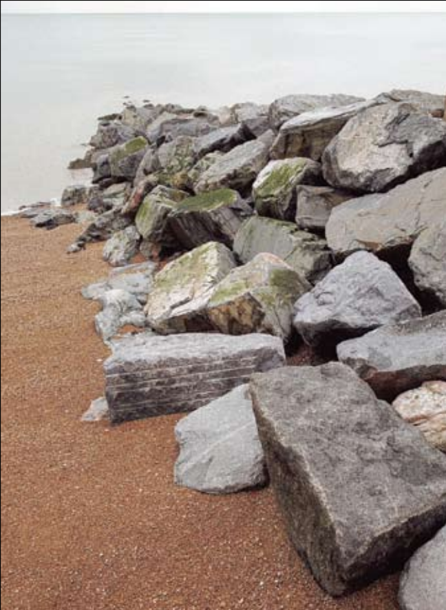
New stone groyne for coastal protection
