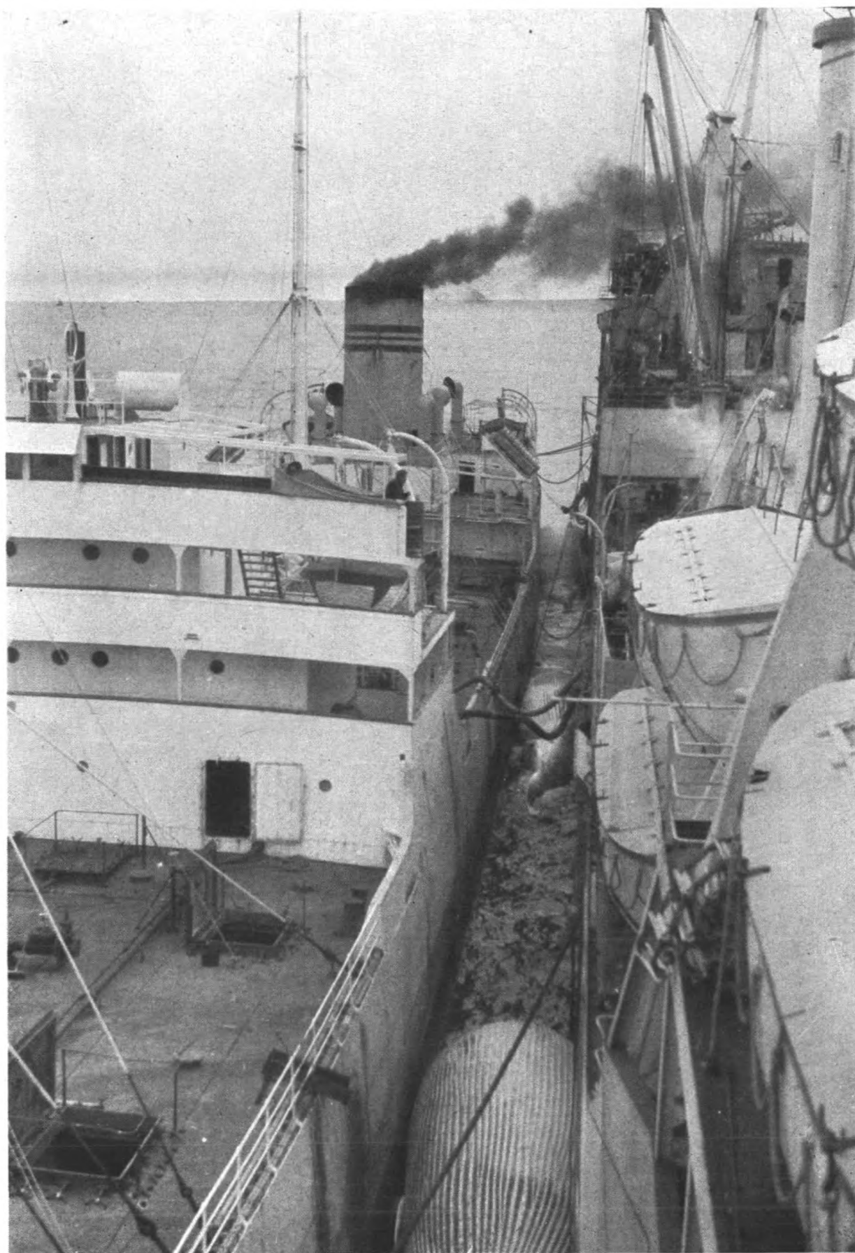
Tanker alongside the floating factory, in January, receiving our first oil production for shipment home. Notice the three whales inflated with compressed air and used as fenders.
