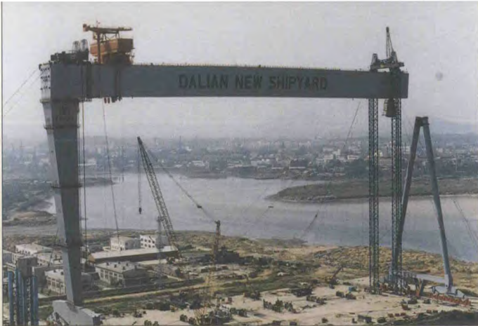
Forecasts were provided to the Dalian shipyard in China to assist the lifting of a 3450-tonne, 182-metre crane gantry into position.
